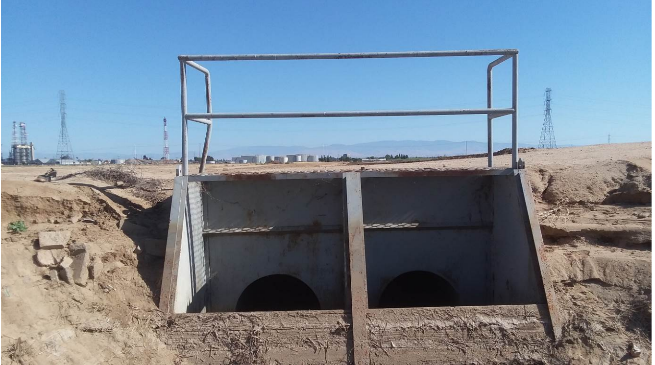
Figure 13 P-15-017237, Beardsley Canal. Dual Siphons and Rail, View to the South
